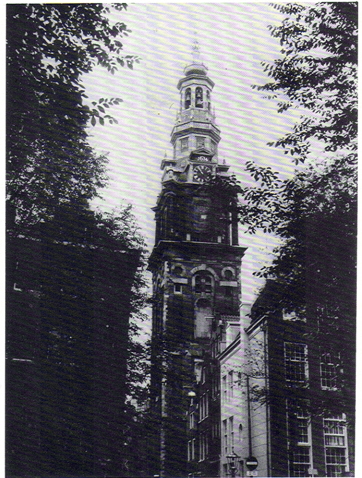
Fig. 14. The "South Church" steeple. The building never reveals itself as a whole except from the inside.
