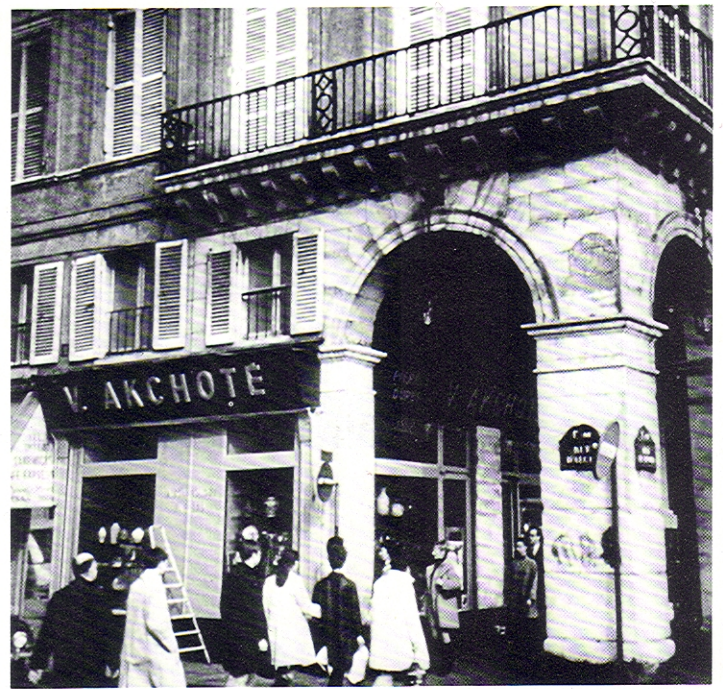
Fig. 17b. Rue de Rivoli. Note the entresol which continues inside the arcade—formal use of a vernacular element.
