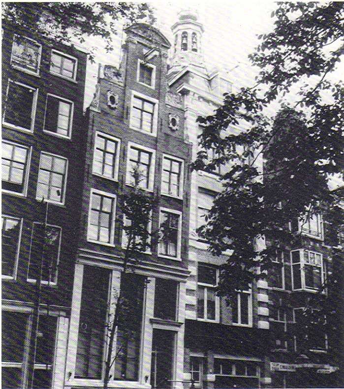
Fig. 3. The facades of canal houses are curtain walls suspended on a structure of brick party walls and wood beam floors, lending themselves to change over a period of time.
